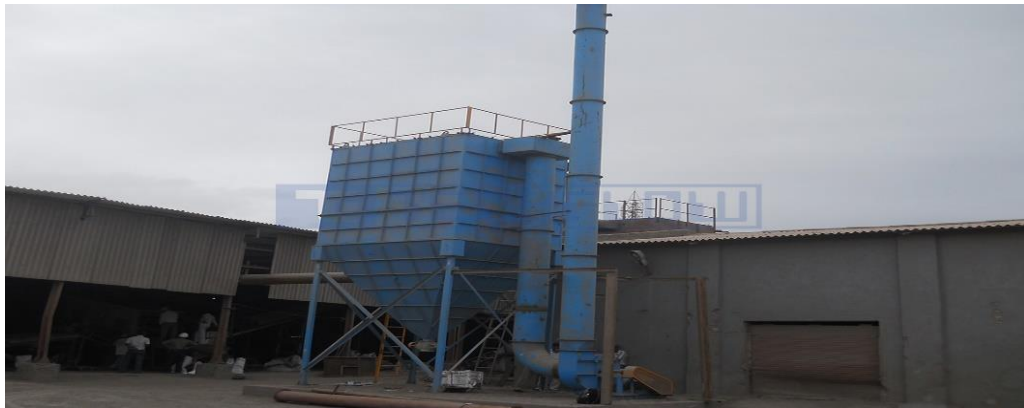
Figure.4. Dust suction and filtration unit (Tech flow, 2002).
